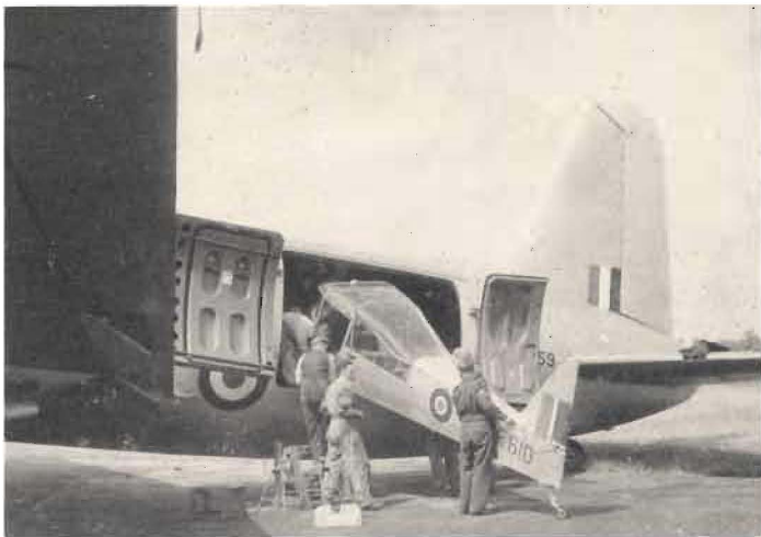
The Auster fuselage being manhandled into the fuselage of the Valetta.
